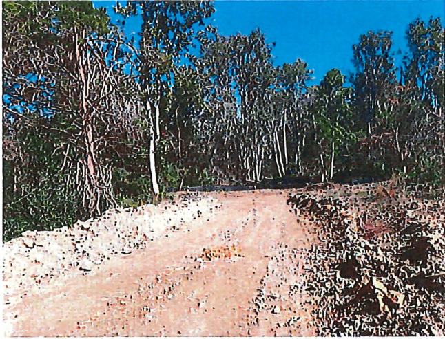
Utility work to be blocked off and Seeded
