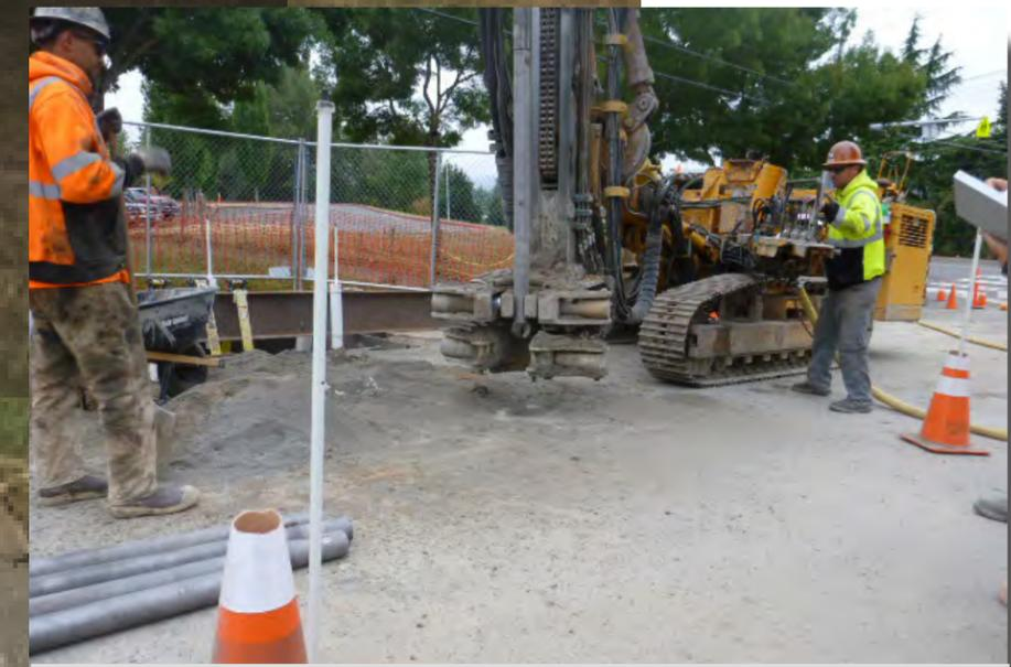
Photo: Construction workers drill bore holes for exploration and to inject filler materials.
