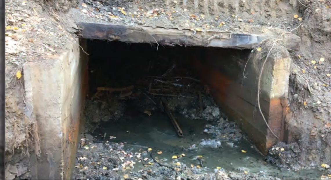
Photo: A collapsing portal to the Dessecker Mine in Ohio.
