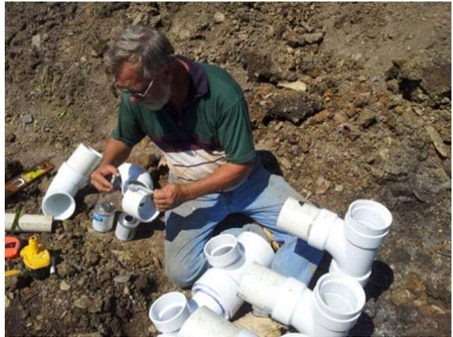
A primary objective was to construct a trompe using inexpensive and readily available materials. Bruce Leavitt, PE, PG assembles a triple-inlet trompe using standard PVC plumbing parts.
