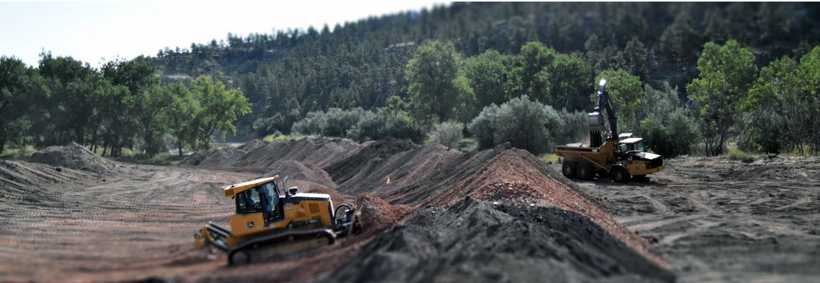
GPS-assisted equipment excavate approximately 47,500 cubic yards of material at the Bair-Collins Mine Reclamation and Floodplain Restoration Project in Roundup, Montana. Photo courtesy of Montana Department of Environmental Quality.
